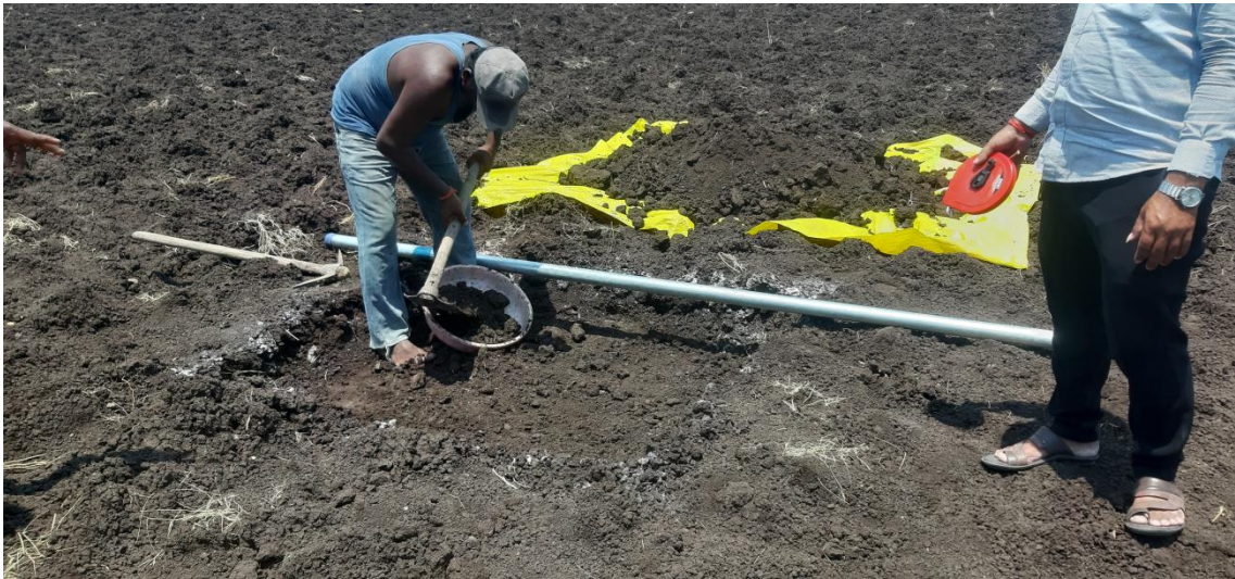
Fig. 2. Digging of pit and heave of soil from pit
