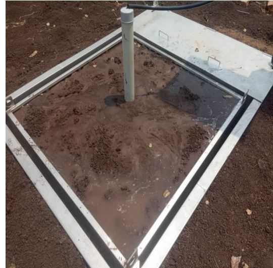
Fig. 15. Saturated Lysimeter after successful installation and calibration
