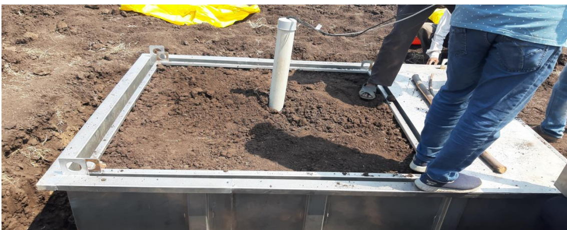
Fig. 12. Completion of Soil filling in the inner tank of Lysimeter
