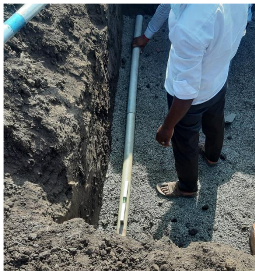
Fig. 6. Levelling the bottom of installation pit
