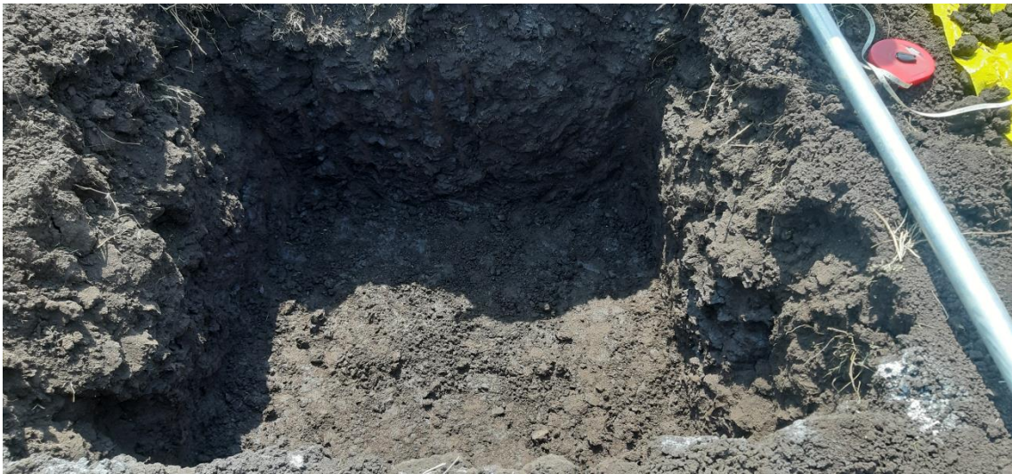
Fig. 5. 1m × 1m pit from which soil was excavated layerwise to fill in inner tank of lysimeter.
