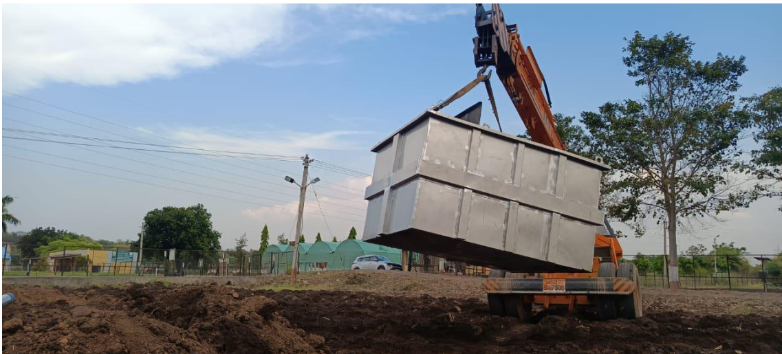
Fig. 8. Transportation of Lysimeter to site
