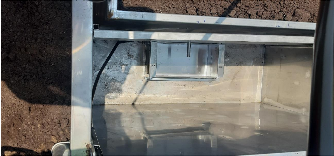
Fig. 13. Placement of Drain tank
