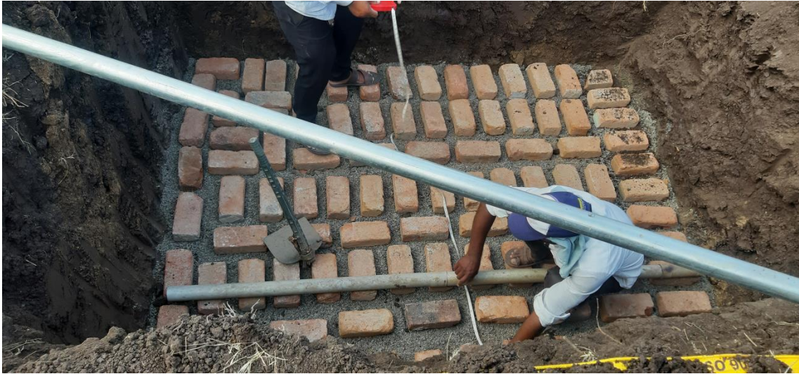
Fig. 7. Bricks foundation below lysimeteras leveled platform
