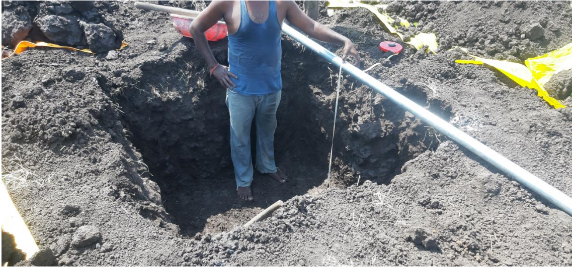
Fig. 4. Measuring the depth of installation pit
